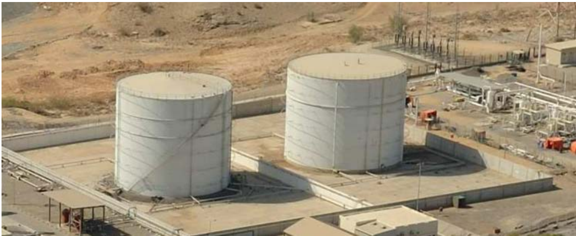
Figure 1: Diesel Fuel Oil Tanks
